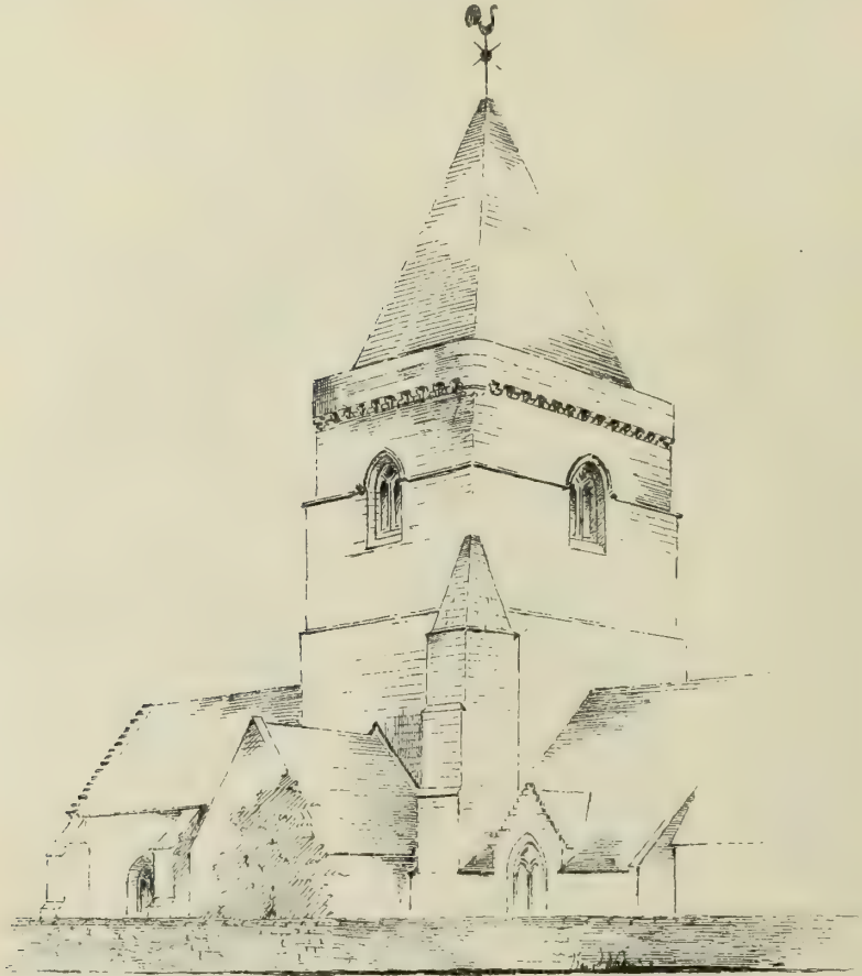
FIG. 1194.—St. Mary's, Whitekirk. The Tower, from North-West.
